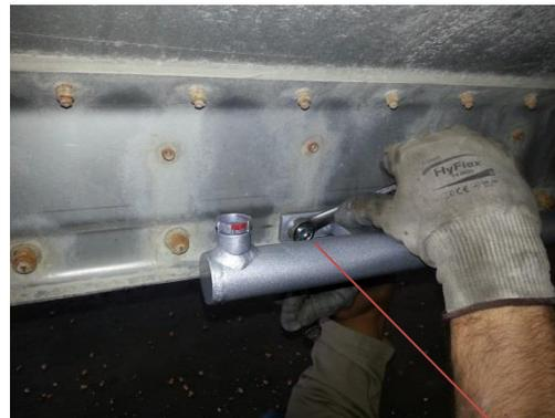
Install the hydraulic cylinders using rollers and provided hardware
